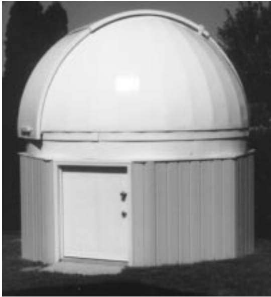
HD10 on House built Octagonal Base Photo Credit: Dave Bair, Hanover, PA
